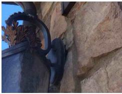
**60:** The garage carriage exterior lights which were believed to have been tested, failed to operate. In many cases, the bulb is usually blown, however, it is recommended that the bulb be replaced and the fixture be tested for proper operation prior to the close of escrow.
