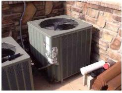
**529:** - We estimate the size of this unit to be 5 tons. This is merely an estimation based on the units model number information. For a definitive size of the condenser, we suggest the buyer employ the services of an HVAC contractor
