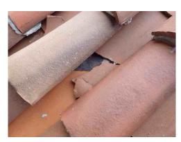
**91:** - There is debris in some of the cricket areas that should be removed to ensure proper drainage.
