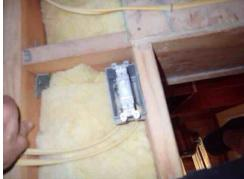
**440:** - Many of the added junction boxes are loose or not attached securely and the wiring was not properly adhered to a solid surface prior to the junction box as per building standard. Improvements are recommended as a safety precautionary measure.
