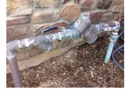
101: - A loop is present and installed at the main water supply for a soft water system.
