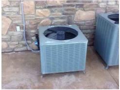
**520:** - We estimate the size of this unit to be be 3 tons. This is merely an estimation based on the units model number information. For a definitive size of the condenser, we suggest the buyer employ the services of an HVAC contractor
