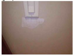
**282:** - Damaged drywall was noted under the basement stairwell and in the theater room. Repairs are recommended and should be conducted by a professional contractor.
