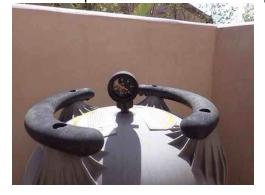
**587:** - The filter grids and backwash valve (if present) are suggested to be inspected prior to the close of this escrow. The grids are susceptible to tears and if damaged will result in a dirty pool/spa. The backwash valve should be tested to ensure it is functional and does not leak.
