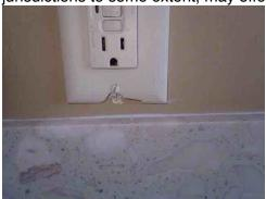
**233:** - There are outlets that are loose or not screwed in tightly when tested at various locations. We recommend that the loose outlets be repaired as necessary to avoid the possibility of future damage or shock - NEC 2014 §406.5.
