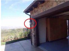
**61:** - The south side exterior light, failed to operate by the switch. In many cases, the bulb is usually blown, however, it is recommended that the bulb be replaced and the fixture be tested for proper operation.
