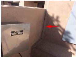
**39:** - There is grout missing from in between the stone facing located at the front wall. Improvements are recommended.
