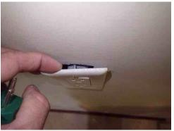
**236:** - There is a gap in the drywall around the cover plate under the stairwell in the basement. Improvements are suggested.
