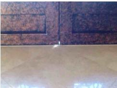
**250:** - There is no hole drilled into the floor for the bottom flush bolt on the stationary entrance door. Drilling a hole is recommended to ensure the door properly latches.
