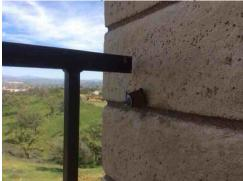
42: - The front wrought iron fence is loose at the footing when pressed upon. Additional stability is suggested.
