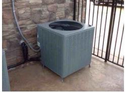
**538:** - We estimate the size of this unit to be 5 tons. This is merely an estimation based on the units model number information. For a definitive size of the condenser, we suggest the buyer employ the services of an HVAC contractor
