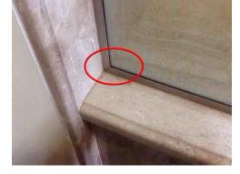
**349:** - Sealant such as caulking / grout is recommended in the shower enclosure at the penetrations to prevent possible moisture entry.
