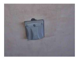
**57:** - There are receptacles at the deck that are missing their exterior cover plate(s). These special type cover plates are designed to keep moisture out of the receptacle replacement of these covers is suggested - NEC 2014 §406.9.
