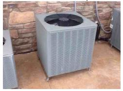
**547:** - We estimate the size of this unit to be 5 tons. This is merely an estimation based on the units model number information. For a definitive size of the condenser, we suggest the buyer employ the services of an HVAC contractor
