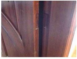
**259:** - We observed screws missing from some of the door hinges. Installing the missing screws is suggested to ensure proper operation of the doors.
