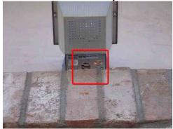
**67:** - The junction box observed at the front west side is suggested to be better sealed at its connection to the building.
