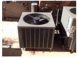
**511:** - We estimate the size of this unit to be be 3 tons. This is merely an estimation based on the units model number information. For a definitive size of the condenser, we suggest the buyer employ the services of an HVAC contractor
