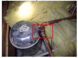
**106:** - Surface corrosion was observed at the copper piping. This is a condition that should be monitored for further corrosion and possible leakage. Future repairs may ultimately be necessary if leaking is discovered. There was no active leaking at the time of the inspection.
