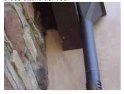
**45:** - The exterior stucco walls appear to show signs of wear which appear to be caused by sprinkler spray. It is recommended that the sprinklers be pointed away from the structure to reduce damage to the structure as a result.
