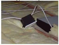
**441:** - There are loose/exposed wires lying in the attic at the time of the inspection. These conductors are suggested to be installed thru conduit for safety and or terminated properly. Improvements are recommended as a safety precautionary measure.
