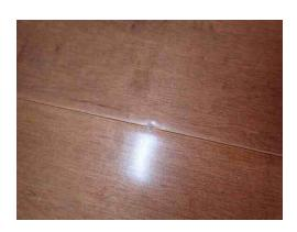
295: - There are damaged tiles in the north end of the first floor hallway.
