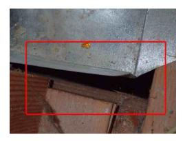
**449:** - The fire stop / fire blocking around the fireplace flue vent is breached by the wiring installed into the chase which is not installed in accordance to manufacturer's / building standards / specifications (and thus leaves a gap) around its perimeter, where it is suggested to be tightly sealed to the top of the ceiling "plates". Further assessment is advised.
