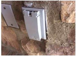
**56:** - Sealant is recommended around the exterior cover plates to wall connections.
