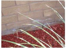
38: - The block wall located at the pool equipment is cracked where attached to the structure.
