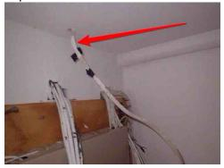
**275:** - The circulator under the sink in the master bathroom is plugged into a receptacle in the closet. The wiring is subject to physical damage in its current state. Improvements are recommended.
