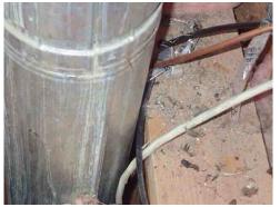
**465:** - The fire stop / blocking is incomplete around the flue vent as pictured, when viewed from the attic. Building code stipulates that fire stop / blocking be placed at every floor level, ceiling / attic or at a minimum of 8 or 10 feet.
