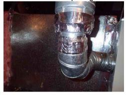
**473:** - The vent pipe has a negative pitch, which could hinder the bi-products of combustion from being vented beyond the residence, and which could contaminate the residence, and should be serviced by an HVAC contractor.
