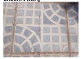
**28:** - The deck does not appear to be properly sloped to shed water and has areas of poor drainage. Furthermore, the drains in the deck are clogged and do not drain properly. Repairs are recommended to ensure proper drainage of the deck.
