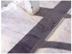
**39:** - The deck does not appear to be properly sloped to shed water and has areas of poor drainage. Repairs are recommended to ensure proper drainage of the deck.
