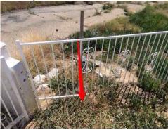
**51:** - The gaps or voids, in the wrought iron fencing are greater than 4 inches which is substandard when a pool, spa or pond greater than 18" in depth is located on the property. IRC 2012 §312.3.
