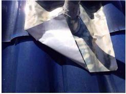
**119:** - There were vent caps which were missing from B vents located at the roof deck. Replacement is suggested to reduce the potential for deterioration or damage to the vent or appliance.
