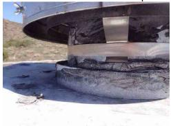
**147:** - Mastic was observed at the base of the flue. This material may not be a listed component of the factory built fireplace system. Further assessment is advised.
