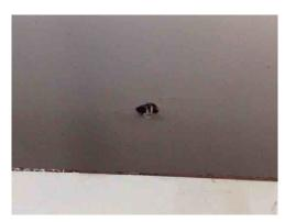
**212:** - The plastic piping penetrates the garage firewall. The point of penetration is suggested to employ a metallic material to maintain the fire rating of the firewall.
