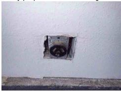
**230:** - Exposed wiring noted, exposed to physical damage or contact was observed in the garage. Wiring which is exposed and within harms reach should be relocated or protected from damage or contact by the use of conduit. An electrical contractor should be contacted for further evaluation and to make any necessary repairs - NEC 334.15.
