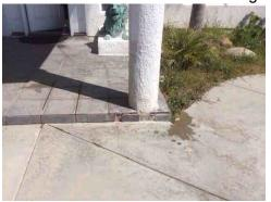
**21:** - The front porch possess a slope which is suspect. The slope may be contributed to settlement. On the other hand the porch may have been constructed in this manner.
