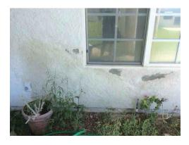
**65:** - Elevated levels of moisture were observed in the exterior walls at the front of the house. This may be due to overspray from the sprinklers or leaking from the decks above.
