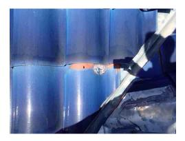
**125:** - Tree contact was noted at the main roof surface. Removal of tree branches and debris is recommended and will reduce wear and tear to the roof covering material.
