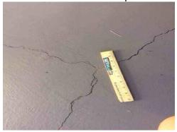
210: - The garage slab does not have any control joints.
