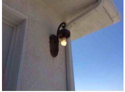
85: - Sealant is recommended around the exterior light fixture to wall connection(s).
