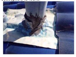
**117:** - There were flashings which were filled with dirt and debris. This material in the flashing pose a potential issue with respect to drainage. The flashing may cause a back up in water run off which may result in a potential leak.
