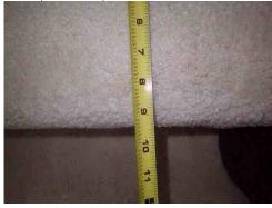
**336:** - The width of the north stairwell appears to be smaller than what current building standards require (3 feet) - 2012 IRC §311.7.1.
