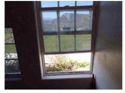
**315:** - The sill in the living room is damaged / cracked and may suggest the drywall has suffered moisture intrusion or damage.
