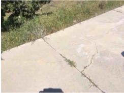
**14: -** The asphalt driveway shows evidence of excessive wear that includes large cracks, raised or settled surfaces, which can accelerate or hasten the life and deterioration of the driveway surface. Sealant and regular maintenance is recommended.
