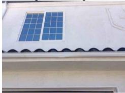
**74:** - The gutters appear to be improperly sloped at various sides of the building which can result in substandard drainage, backup, premature wear, rust, roof leaks and trim damage.
