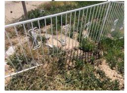
**50:** - The pool barrier is short. The barrier should be maintained at the local minimum building standard height of 60 inches (depending on code in jurisdiction) but this figure should be verified with the local building
