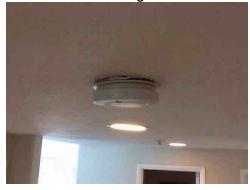
**347:** - The smoke alarm in the downstairs hallway near the laundry room is loose and should be better secured to the ceiling.
