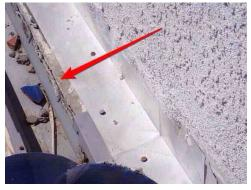
**122:** - The tile membrane does not appear to terminate on top of the valley metal. The membrane should terminate on top of the valley metal to properly shed water into the valley instead of underneath it.
