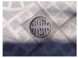
**29:** - Sealant was noted at the deck on the grout joints of the tile and up against the house. This may be an attempt to stop a previous leak on the deck.
