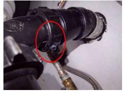
**369:** - The garbage disposal tail piece is loose where it connects to the plumbing. No leaking was observed, however, securing the plumbing is recommended to prevent a leak.
