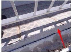
**32:** - Evidence of leaking was observed from underneath the deck and on the exterior walls of the house. We are unable to determine the methods in which the deck is waterproofed without destructive testing. Our fear is that the wood framing members of the deck may be damaged/rotten and in need of replacement. Further evaluation is recommended by a licensed general contractor.
