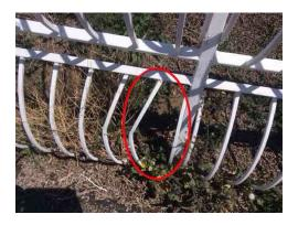
**52:** - The bottom and / or sides of the fence / gate exceeded the minimum allowable space of 2 inches over grade for barriers which lead to a pool yard. This applies to fencing and gates alike. Repairs are suggested to adhere to the safety provisions set forth by the local building authority - 2012 IRC §AG105. Local code is likely more restrictive.
