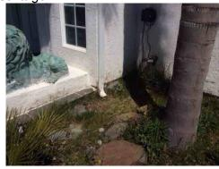
77: - There are downspouts that are too close to the ground and should be raised at least 6 inches for maximum flow.
