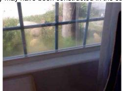
**314:** - Sash cords / balancers (the ropes that hold up the windows) are inoperable on the window(s) in the garage. Repairs are suggested for proper operation of single and double hung windows and should be performed by a professional contractor. All of the inaccessible single hung windows are suggested to be tested once they are made accessible and prior to the close of escrow.
