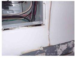
**255:** - We observed openings within the service equipment panel. Openings in the panel are not suggested and should be closed or sealed off by a professional contractor.
