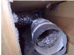
**358:** - The gas dryer vents incorrectly through a return-air compartment. This could contaminate the return-air compartment with the bi-products of combustion, and the should be isolated or rerouted. We fell it prudent to note that there is in fact an isolated return air duct which may or may not allow contamination of the interior if such a leak of the dryer duct exists.
