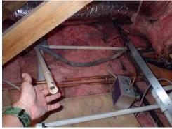
**482:** - The condensation pan appears to be severely rusted and deteriorated. A rusted pan may suggest a leaking secondary condensate drain, leaking primary, switched condensate drains or leaking "A" coil. In light of this finding, we suggest the buyer have an HVAC contractor evaluate the pan.
