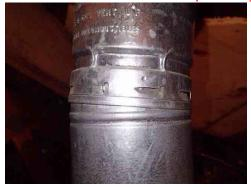
**472:** - The vent was wrapped in a metal tape therefore, the vent was not fully visible for inspection. Vent piping is suggested to be tightly assembled therefore not needing any auxiliary sealant such as tape. Furthermore, many manufacturers do not approve of the installation of this material on their venting systems as a means to seal openings.
