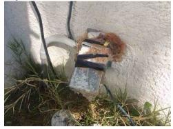
**81:** - All of the exterior ground-fault protected outlets did not trip or are not protected upon test, and should be replaced.
