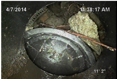
4/7/2014 11:38:18 AM Sewer line not connected at guest house
