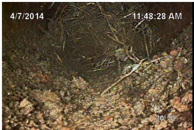
4/7/2014 11:48:28 AM Root intrusion and possible collapsed pipe
