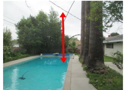
electrical service conductors too close to pool surface
