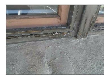
1.34 - Sealant is needed at various areas around the exterior trim to exterior wall connections as preventative maintenance and to prevent the possibility of moisture penetration or damage.
