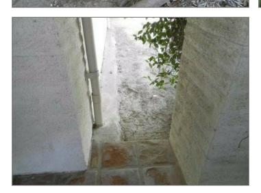
2.6 - Planters were observed close to the foundation. Without proper drainage and sealant at the exterior wall, these planters hold moisture / soil close to the exterior wall covering and foundation which may result in damage
