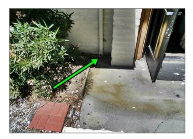
1.41 - The front gutter was found to be sagging, which will cause the water to pool in the gutter, resulting in more sagging, or possibly, damage to the gutter. Additional support is recommended to help secure the gutter to the fascia.
