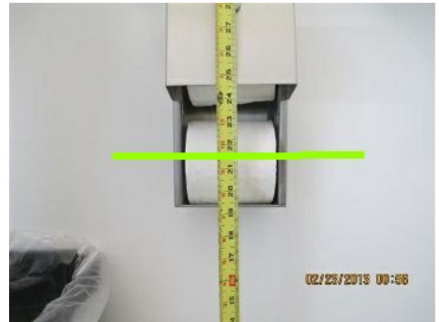
toilet paper roll too high
