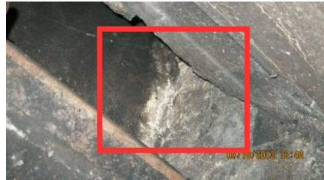
missing mortar
