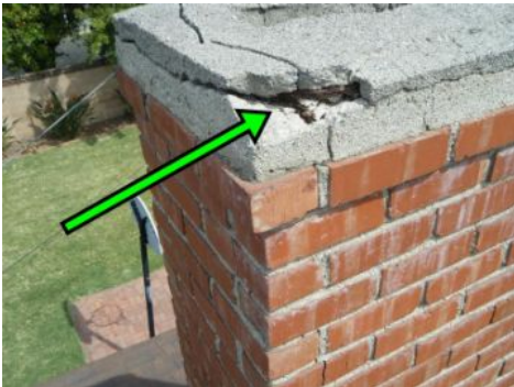
damaged crown
