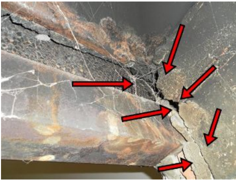
missing mortar
