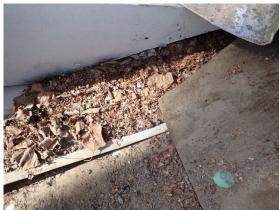
**11:** - We observed the use of roof cement against the side of the pan metal. This installation may trap water under the metal and not allow it to properly drain. Removing the roof cement is recommended.
