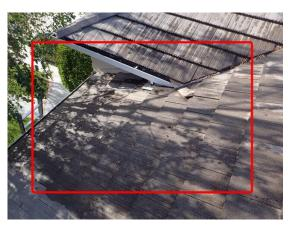
**17:** - The membrane at the bottom edge of the roof appears to be deteriorated and is suggested to be repaired.
