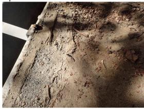
**18:** - Water appears to be backing off of the valley metal and deteriorating the membrane due to the debris in the valleys which may be keeping the water from properly draining. Cleaning the valleys and replacing the membrane is recommended.
