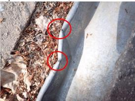
13: - There is a nail at the bottom of the pan flashing that is suggested to be sealed.
