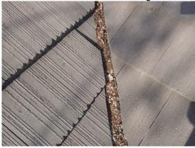
**10:** - There are flashings that are filled with dirt and debris. This material in the flashing pose a potential issue with respect to drainage. The flashing may cause a back up in water run off which may result in a potential leak.
