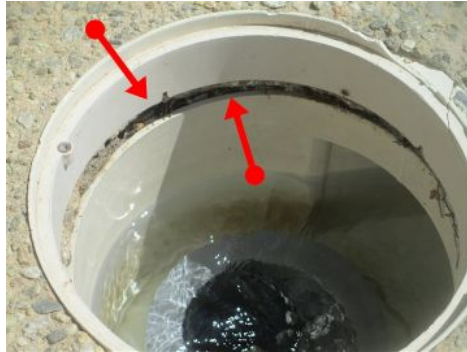
sealant is suggested within skimmer
