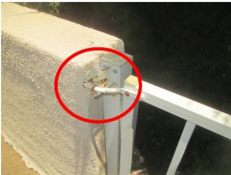
gates to pool yard do not self latch
