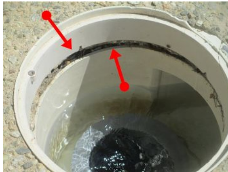
sealant is suggested within skimmer
