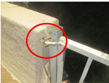
gates to pool yard do not self latch
